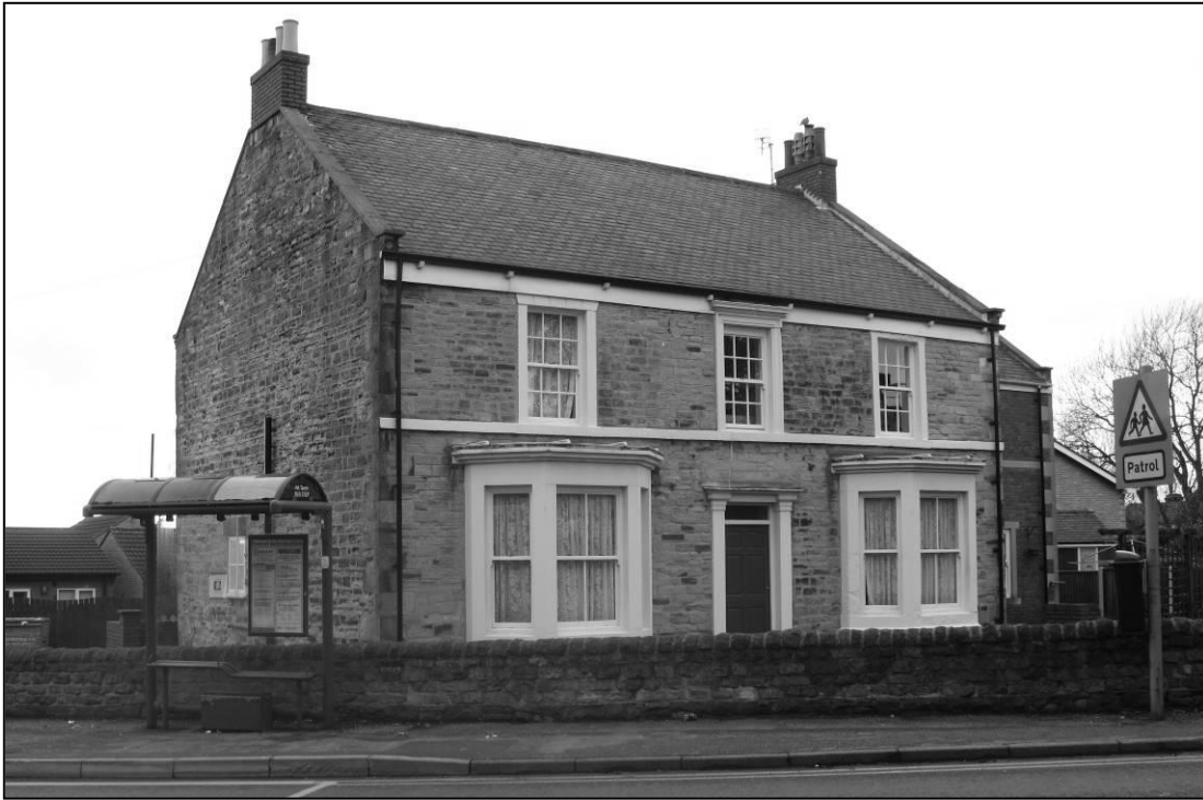
The 1970s renovation, though extensive, was an obvious success, as this January 2010 view of Sutton Lodge shows. Now officially known as 'Sutton Court Lodge' this building currently provides personal care and support for seven people with learning disabilities. The service is provided by Enable Care and Home Support Ltd.
